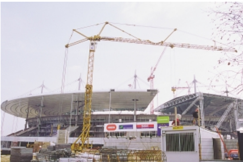
Tower crane or wind turbine slewing movement.
