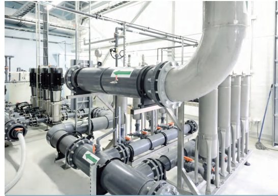
Municipal water supply
